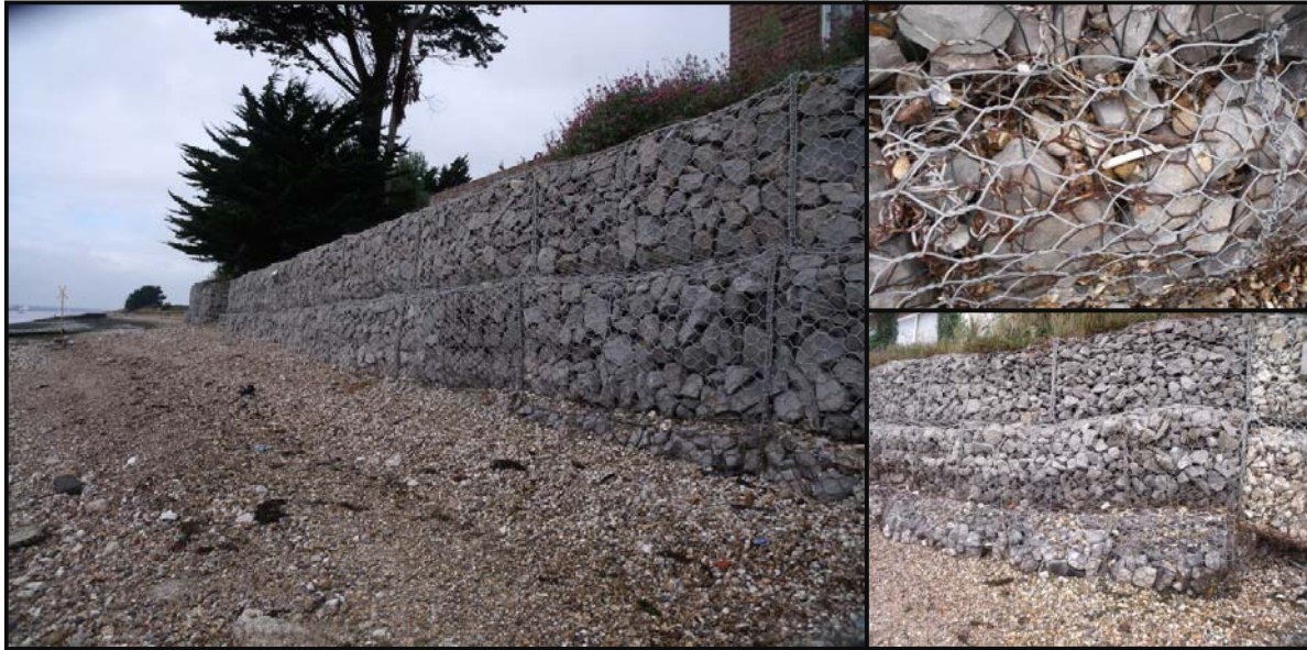
Figure 10: general arrangement of Defence Length 9, including detailed images of mass concrete pours and gabions
