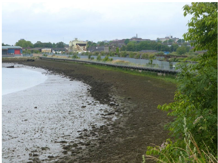
Figure 20 - Boardwalk in Southampton
